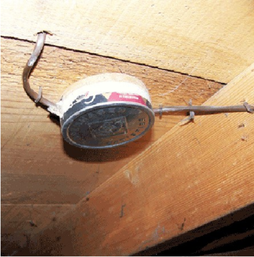
Dip can j- box, from good ole boy engineering and power wiring installers Inc.
